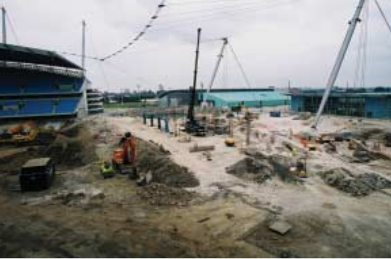
5. left: Removal of temporary seating, 2 September 2002.
